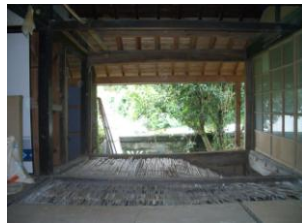
Figure.8 Rotten floor
