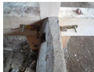
Figure.17 Reinforcing metal of column base
