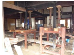
Figure.10 Level adjustment (Japanese-style room)
