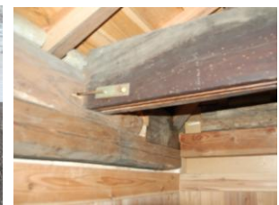
Figure.18 Reinforcing metal of column's top
