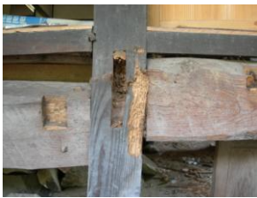
Figure.7 Rotten pillar
