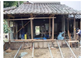
Figure.11 Level adjustment (Kitchen)
