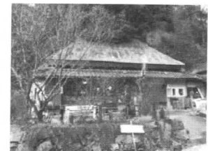
Figure20. Exterior of the House Renovated by a Tenant
