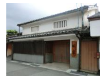
A renovation of a private house located with a hospital
