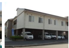
Facility E Photo.9
