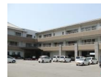
Facility B Photo. 8
